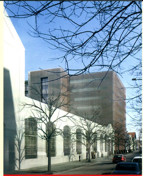
Karlin Halls, Prague 8 ■ Source: AED project
