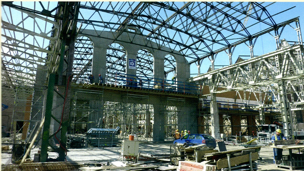
Karlin Hall 1 – under construction ■ Investor: Zdeněk Bakala Group
