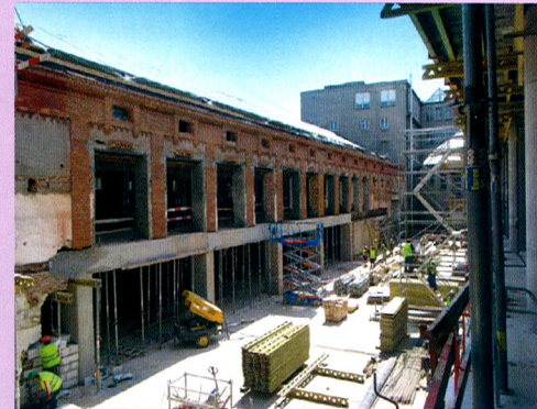
Breda & Weinstein Opava – under construction
